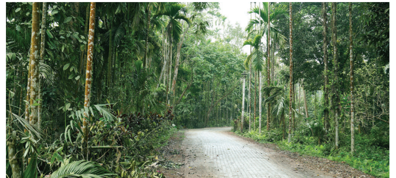
Newly paved road, cycle stand and street light in Katoni Gaon
