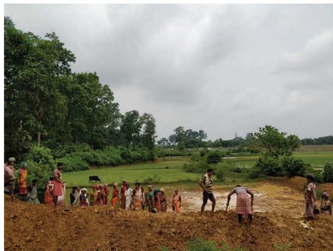
MGNREGS work in progress, Matabari block, Gomati
